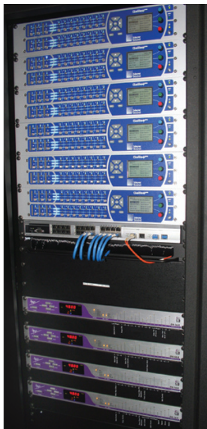
Meyer Galileo and Apogee DA-16X drive rack
